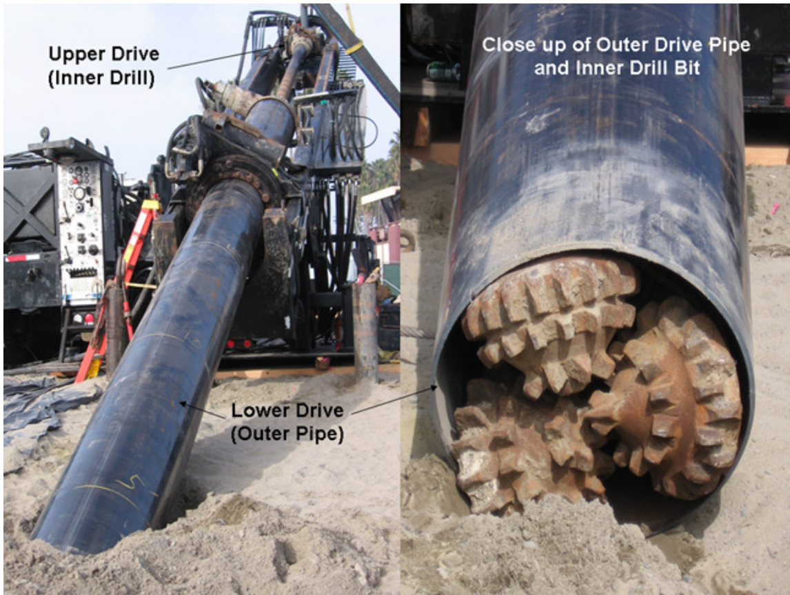
Figure 8 – Dual Rotary Well Construction
